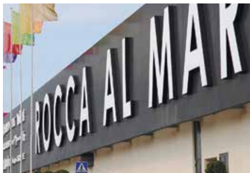
Rocca Al Mare shopping centre facade
