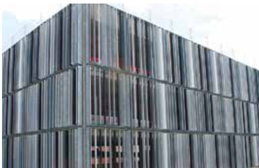
Car Park facade
