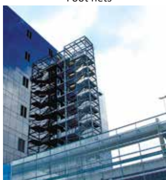
Delta Plaza Tallinn car park facade
