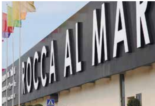
Rocca Al Mare shopping centre facade
