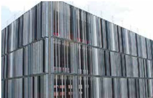
Car Park facade
